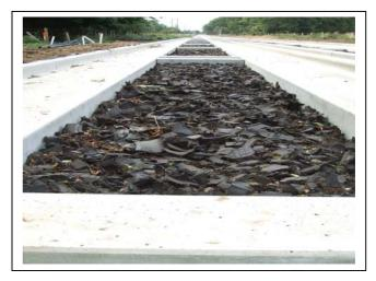
The photos above show: (top left) a beam being lifted onto the Terberg, (top right) two guided buses on the track, (bottom left) a guided bus on the track (bottom right) shredded tyres in between the tracks.
