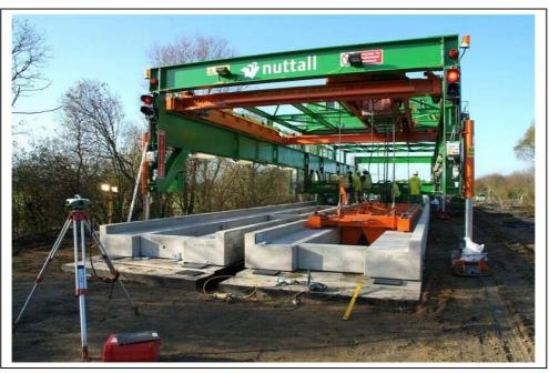
The photos above show: (top) the concrete beams used for the track, (bottom) The Gantry machine laying the beams.
