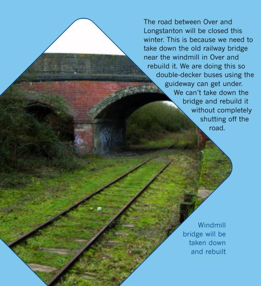
The diversion route is through Willingham on the B1050 and Over Road. The new bridge will be completed and the road re-opened by June 2008. When the bridge is being taken down and rebuilt we will protect the wildlife site in Over cutting.
