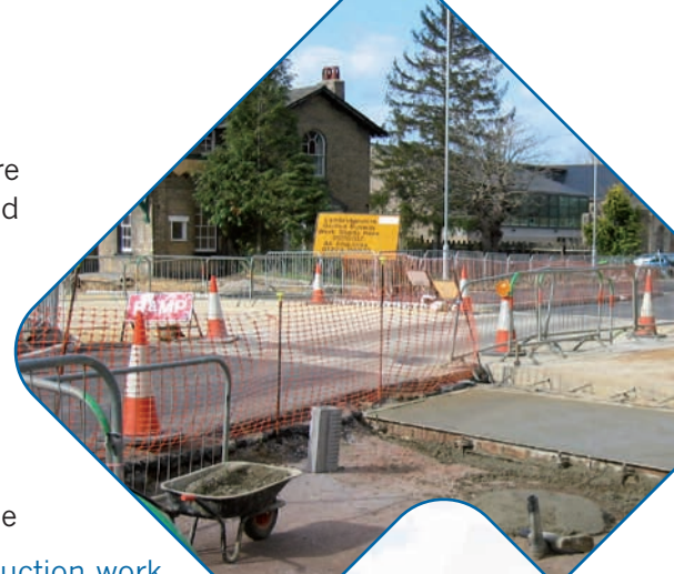
Construction work at Station Road, Histon/Impington
